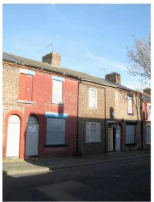
The buildings have clearly not been maintained for a considerable time, and certainly since they were boarded up. As ever in this situation their condition will deteriorate rapidly, particularly where water penetrates the structure and which will affect both timber roof and upper timber floors.
